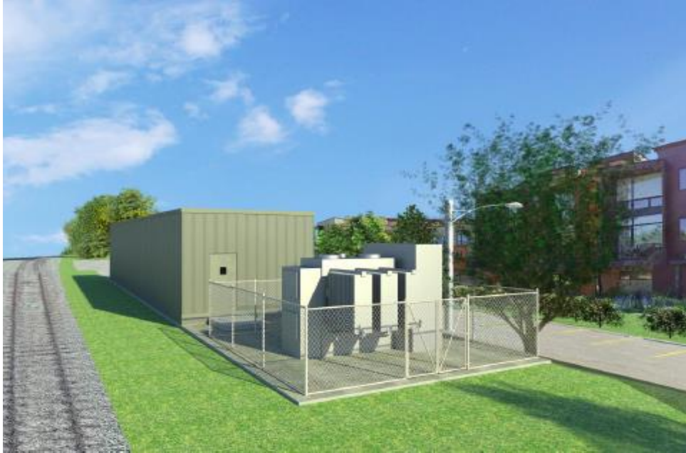
View from Southwest (Trackside)
