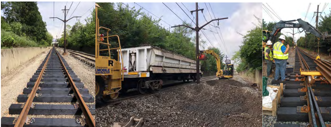
Figure 61: Light Rail Ongoing Track Rehab
