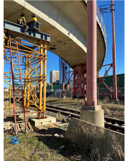
Figure 47: Jacking Process on the Waterfront Line Bridge
